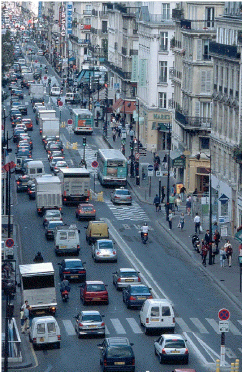
Figure 16 : Bus lane on Rue de Rivoli. Its width is 4.5 m. It is physically separated from the other lanes by a curbstone.
